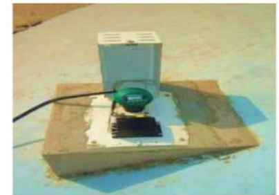
Installation at KAHODA, GJ
