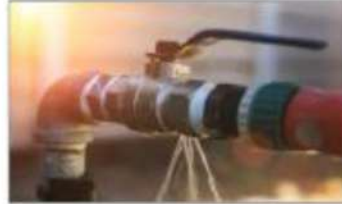
Smart Water Leakage And Flow Schedule Prediction
