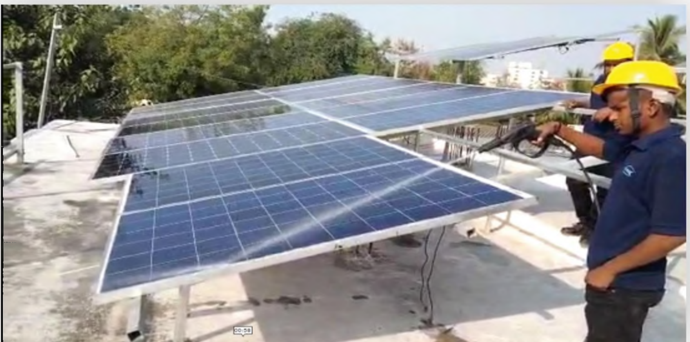
Panel Cleaning with Jet Spray
