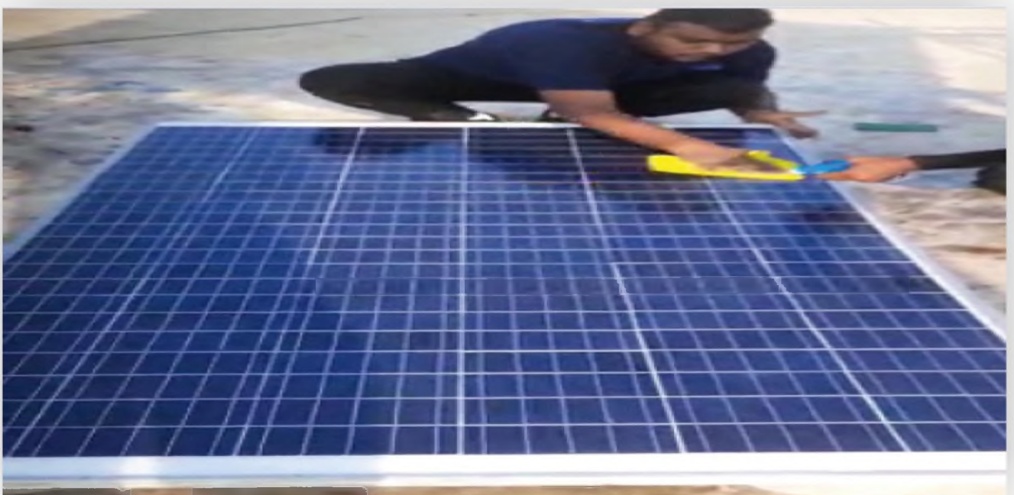
Panel Cleaning with Coating
